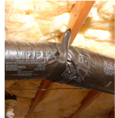
Duct sealed and insulated.
