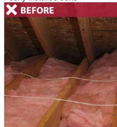
Poorly installed batts
