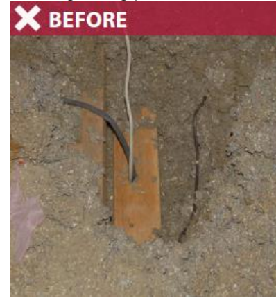
Leaking wiring penetration
