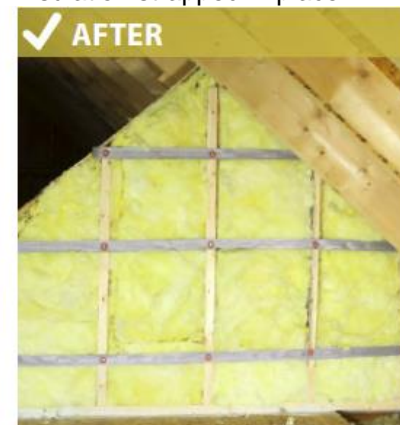
Insulation strapped in place
