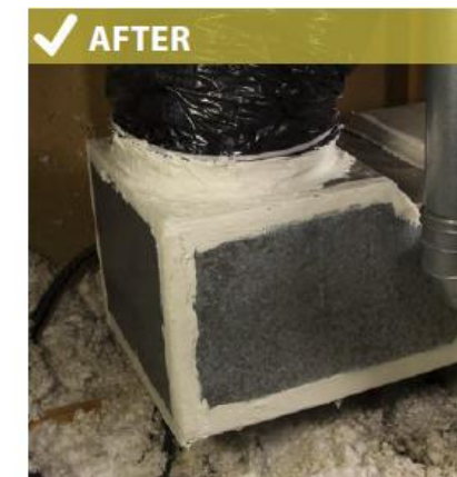
Duct and plenum sealed
