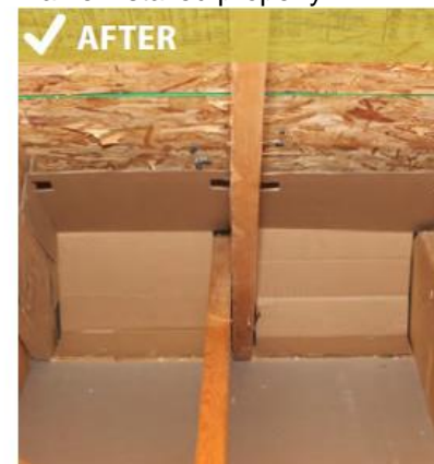
Baffle installed properly
