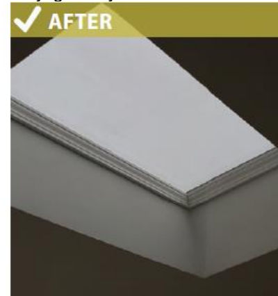
Skylight fully air sealed
