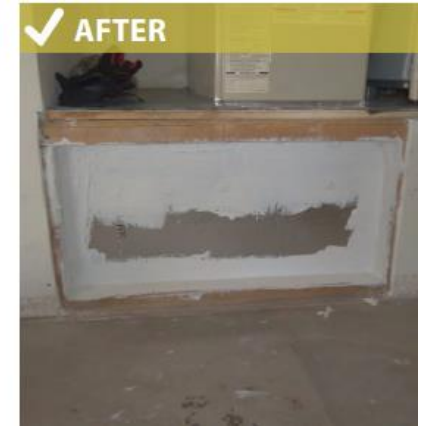
Platform lined and air sealed
