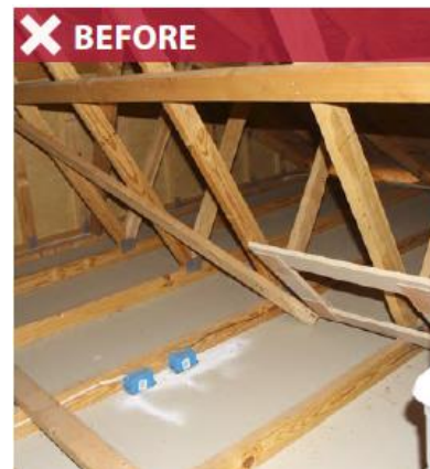
Attic without insulation
