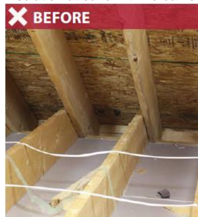
Insulation at eave with no baffle
