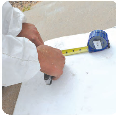
2. Cut blocking material to fit
