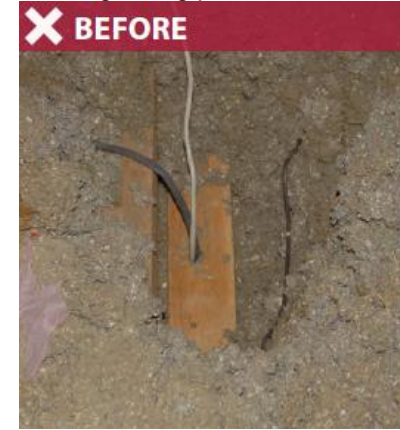
Leaking wiring penetration
