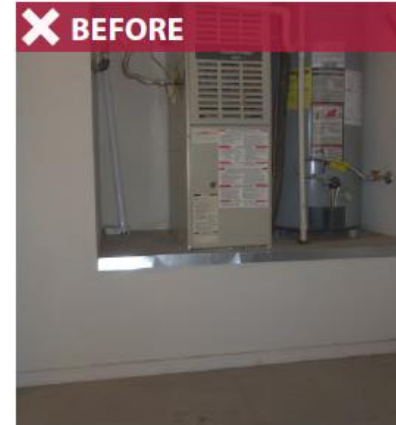
Rough frame support platform
