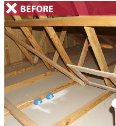
Attic without insulation
