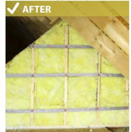
Insulation strapped in place
