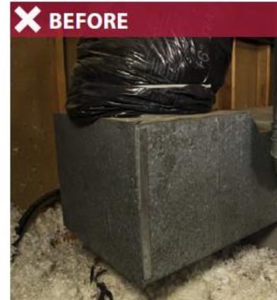
Duct and plenum not sealed
