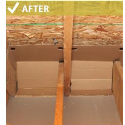
Baffle installed properly
