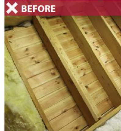
Unsealed tongue & groove ceiling
