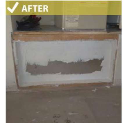
Platform lined and air sealed
