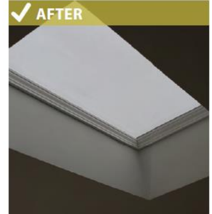
Skylight fully air sealed
