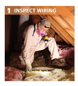
Use non-contact testing method to identify live wiring.
