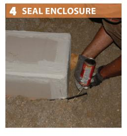
Finished air tight enclosure. No insulation on top.
