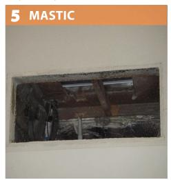
Install rigid duct support material that is at least 1 inch larger than the hole.
