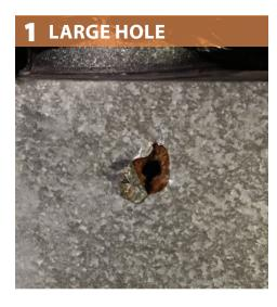
Install rigid duct support material that is at least 1 inch larger than the hole.
