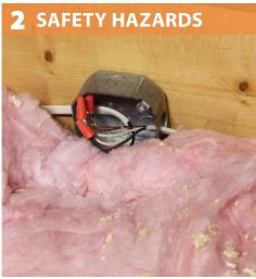
Install and seal blocking as needed to contain dense pack insulation.
