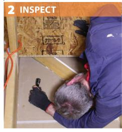
NOTICE: Do not insulate cavity until safety hazards are corrected (e.g., flue pipes, uncovered junction boxes, etc.).
