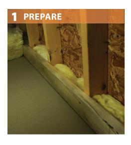
Cover or fill cavity at ceiling height with rigid material. Fasten as needed.
