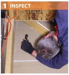
Do not insulate cavity until safety hazards are corrected (e.g., flue pipes, electrical issues, can lights, etc.).
