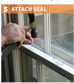
Attach a foam strip to the bottom of the sash.
