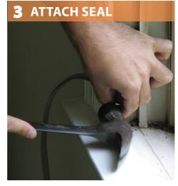
Cut the v-seal to fit on the back side of the top of the sash.
