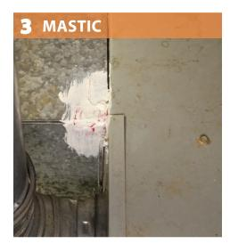
Apply fiberglass mesh tape to completely cover and extend beyond mastic.
