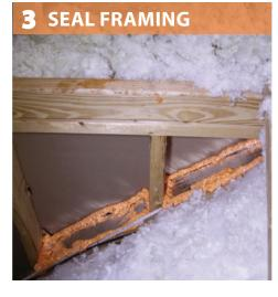
Reinstall batt insulation in full contact with all sides of cavities without gaps, voids, compressions, misalignments or wind intrusions.
