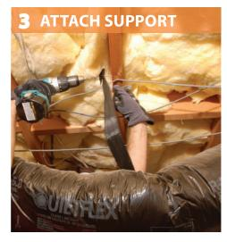
Flex duct supported every 4' having no crimps or interior dimension reduction.
