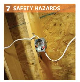
Maintain minimum of 3-inch clearance from soffit vents.
