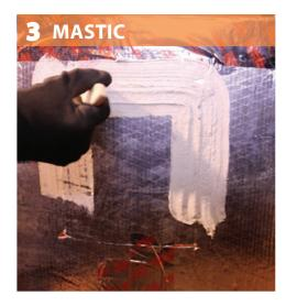
Apply fiberglass mesh tape to completely cover and extend beyond mastic.
