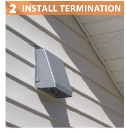
Install duct pieces with crimped ends pointed in the direction of air flow. Cut pieces to fit.
