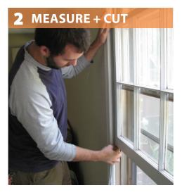
Raise the sash and stick the weatherstripping to side jambs. Tack in place at top and bottom.
