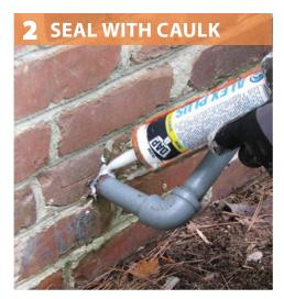
For holes 1/4 in. to 3/4 in., install backer rod, copper mesh and seal with water-proof caulk.
