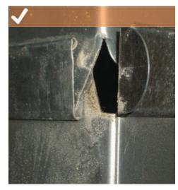
Take Off Collar to Plenum: Gain access to joint by removing outer nylon tie band or tape and peeling back insulation.
