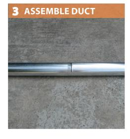
For the connection between the duct and the termination, install the termination cap adaptor.
