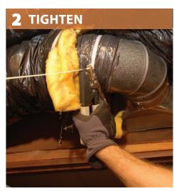
Cut off tie ban tail using tie band tensioning tool.
