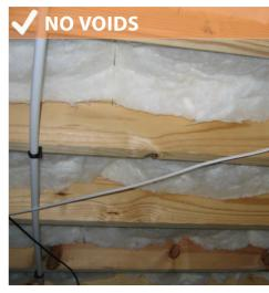
Install insulation to completely fill floor and/or cantilever framing or to maintain permanent contact with the subfloor.
