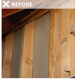
Knee wall with both a top and bottom plate and air sealed.
