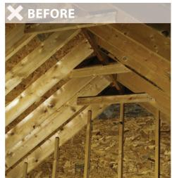
Radiant barrier installed only at the roof deck.
