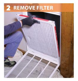
If present, score any mastic or duct tape sealing between return grill flange and return. Remove screws.
