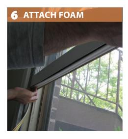
Temporarily seal the top sash using a removable sealant.
