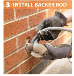
For holes greater than 3/4 in., use hydraulic cement to seal penetrations.
