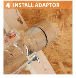
Fasten duct connections with a minimum of three equally spaced screws.
