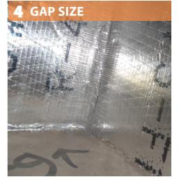
Seal all gaps, seams, holes and penetrations with UL181M mastic.
