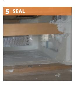
If refrigerant and condensate lines penetrate the platform return, seal with mastic and provide infill as needed.
