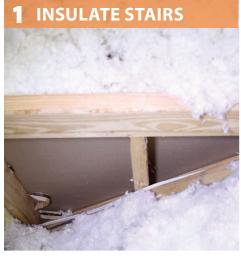
Fasten rigid material to ensure batt insulation stays in place and seal all
