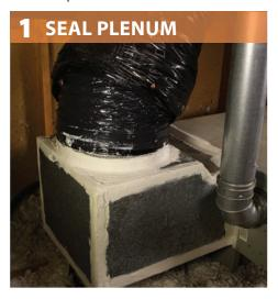
Peel back outer liner and insulation.
