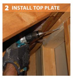
Air seal joints, cracks and penetrations including connection between interior surface and framing.
