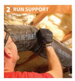
Attach support material to framing (i.e., truss, rafter or joist).
