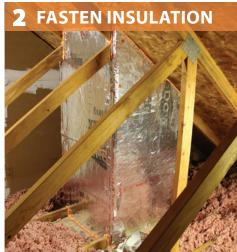
Air seal all seams, gaps or holes as well as roof deck and ceiling connections.
