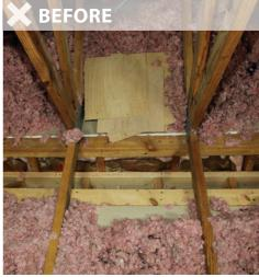
Wall cavities capped and air-sealed.
