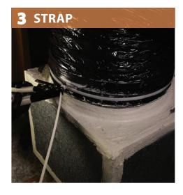
Seal inner liner with mastic. Choose the appropriate sealing technique based on hole size.
