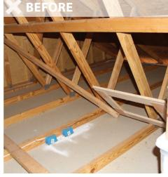
Finished attic adequately marked for insulation depth
