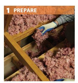
If insulation is on exterior wall, cut at ceiling level.
