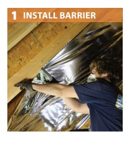
Apply radiant barrier to gable walls while maintaining ¾-inch air space. Radiant barrier should not block gable vents.
