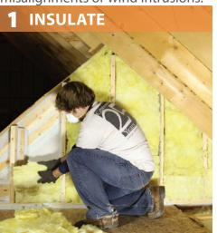
Fasten non-rigid material to ensure batt insulation stays in place.
