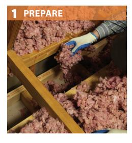
Install support material (e.g., 2X) for spans wider than 24 inches.
