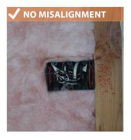
Install insulation to completely fill floor and/or cantilever framing or to maintain permanent contact with the subfloor.
