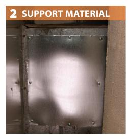
Apply a coat of mastic to completely cover and extend beyond support material.
