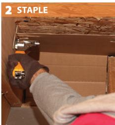
Baffle installed to the exterior side of the top plate to allow for the highest possible R-value.
