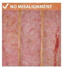
Install insulation to fill the cavity between conditioned and unconditioned space without gaps, voids, misalignments or compression.
