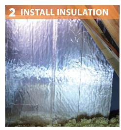
Air seal all seams, gaps or holes in, or adjacent to, foam sheathing. Provide infill as needed.
