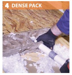
Install and seal blocking as needed to maintain dense pack insulation.
