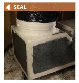
Replace outer liner and insulation.
