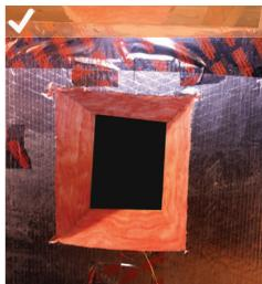
H. Panned Returns: Create temporary access hole by cutting hole through accessible area of return.
