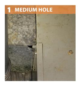
Install temporary tape over seams, cracks, joints, holes and penetrations.
