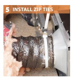
Seal each flex duct connection with mastic.
