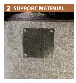
Apply a base coat of mastic to completely cover and extend beyond support material.
