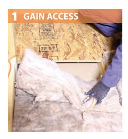
Inspect along and beneath platform for possible safety hazards (e.g., flue pipes, uncovered junction boxes, etc.).
