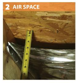
Install radiant barrier to separate attic above conditioned space from adjacent attics. Should be installed to withstand local wind loads.
