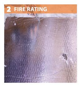
Install and fasten rigid sheathing over stairwell.
