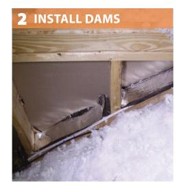
Seal all gaps, holes and seams in adjacent framing at top of stairwell.
