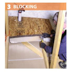
Fill cavities to recommended density for material.
