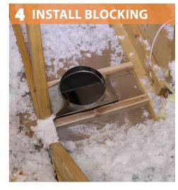
Mechanically fasten, support and seal flex duct to both boots.
