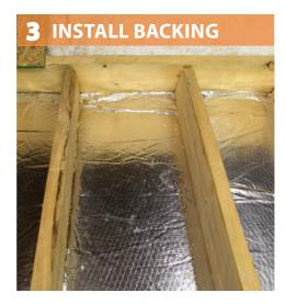
Air seal backing using a sealant that meets fire barrier specifications.
