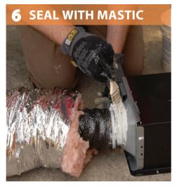
Pull flex duct insulation into place and seal with mastic.
