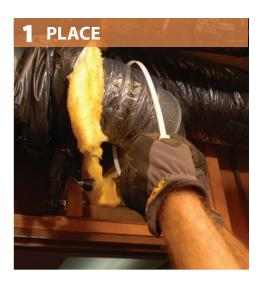
Tighten tie ban using tie band tensioning tool.
