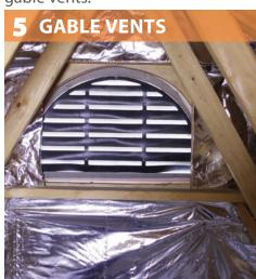
Maintain air space no less than <sup>3</sup>/<sub>4</sub>-inch between barrier and bottom of the roof deck.
