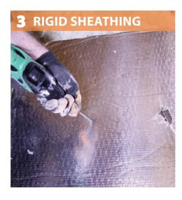
Air seal all gaps, holes and seams of rigid sheathing.
