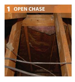
Install cap to cover entire chase. Install support material as needed. Fasten in place.
